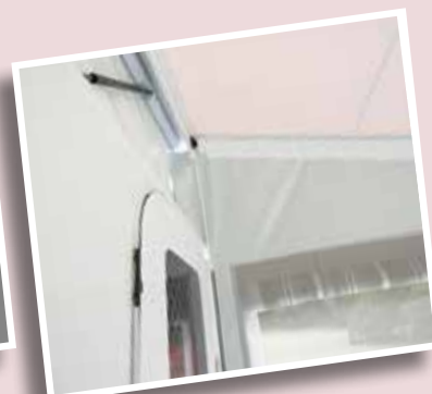
Glued on Poptop flap to Kakadu walls
